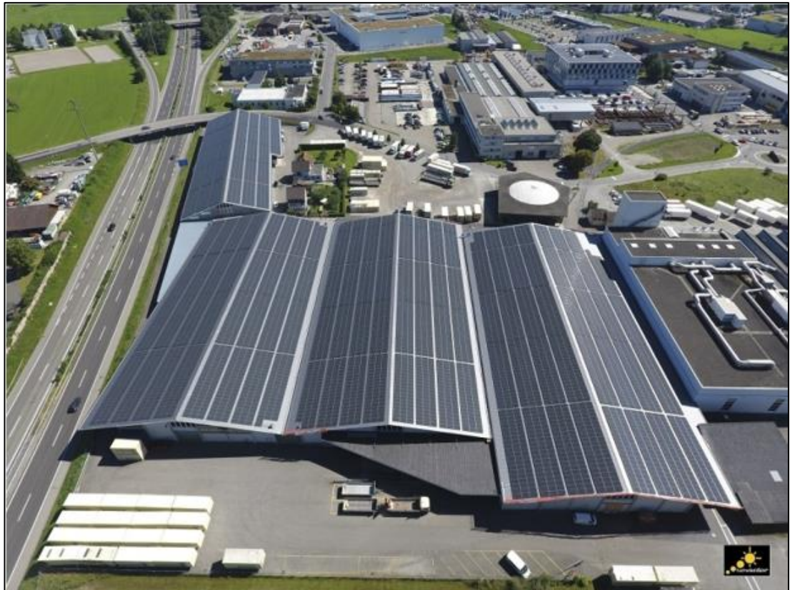
Figure 2.1. Rooftop PV system of a Swiss logistics firm, Switzerland [59].
