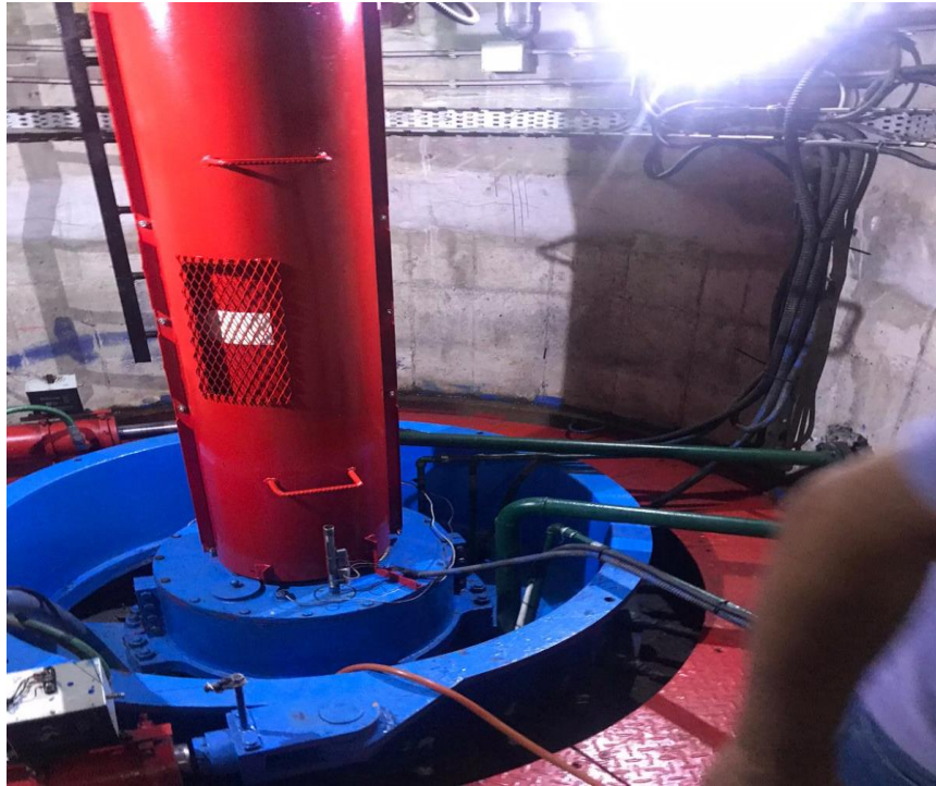
Figure 3.1. Kaplan turbine.
