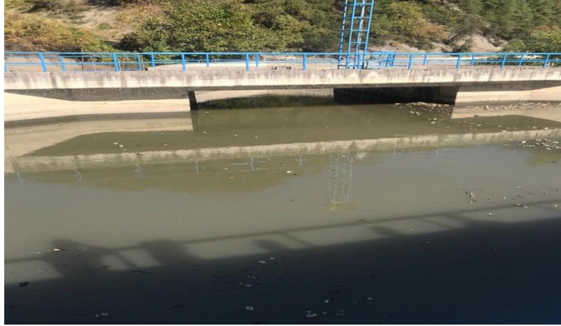
Figure 4.3. Forebay of RRHPP.
