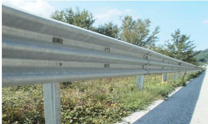
Figure 3.4. Thrie beam guardrail [15].
