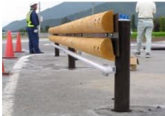
Figure 2.1. Steel post timber barrier [56].
