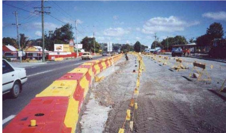
Figure 3.16. Plastic barrier application [13].
