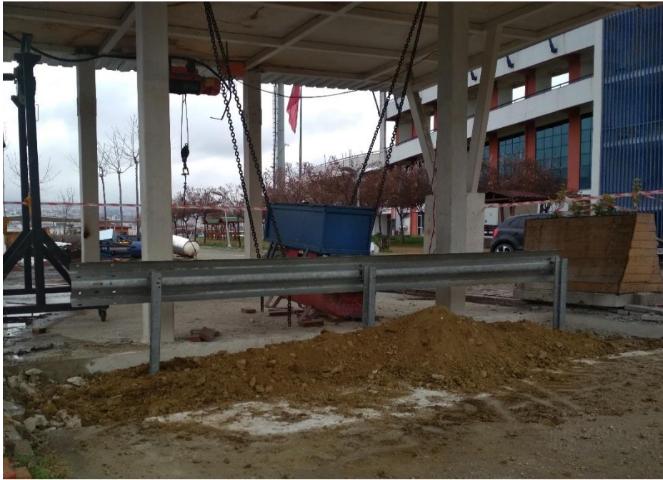
Figure 5.19. W- beam steel barrier after installation process.
