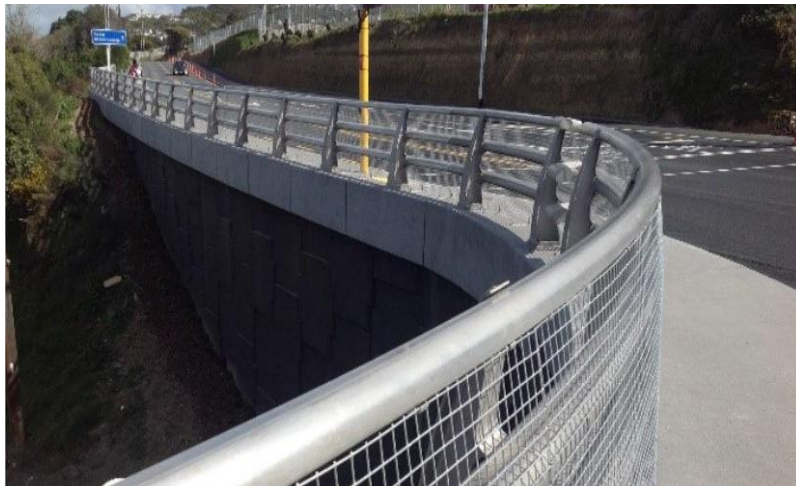
Figure 3.5. Steel tubular bridge barrier [75].
