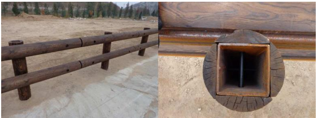
Figure 2.10. Aesthetic timber guardrail reinforced by steel [60].
