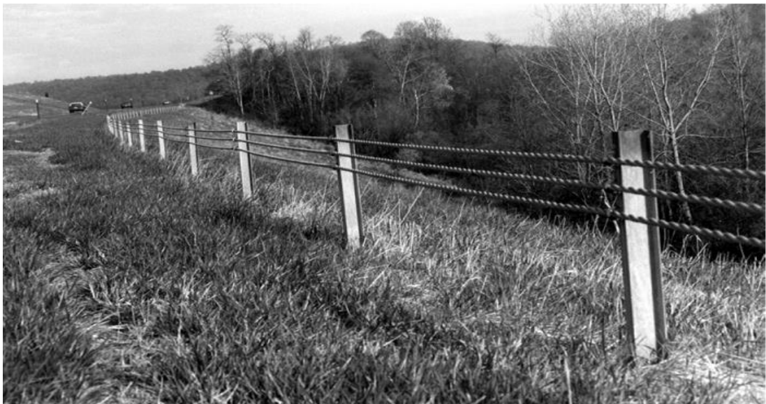
Figure 2.1. Three strand cable barrier [34].
