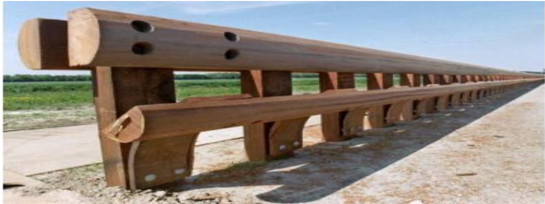
Figure 2.8. Timber guardrail without reinforcing [69].
