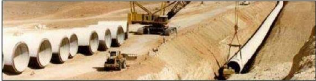
Figure 3.4. Connecting pipe segments Source [83].
