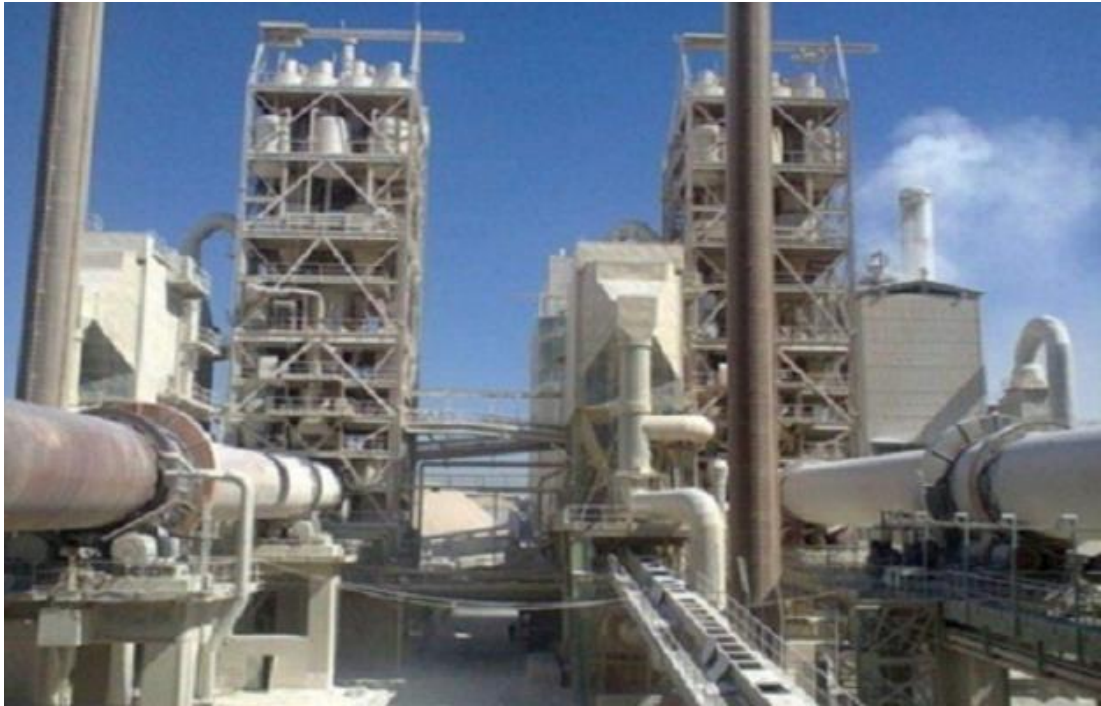
Figure 1.1. Fallujah White Cement Plant.
