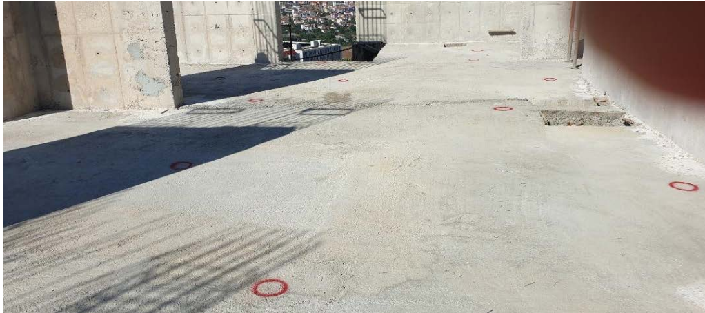
Figure 3. Determining concrete test hammer points
