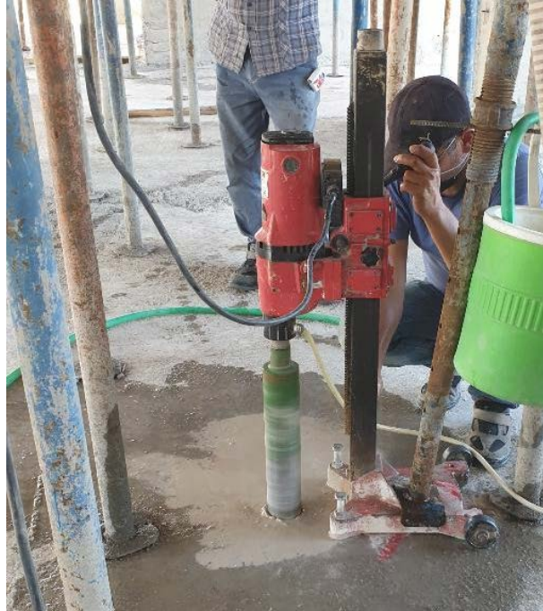
Figure 6. Vertical core application of concrete for a floor slab
