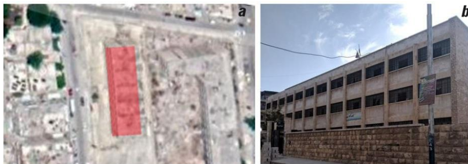
Figure 3.1. a) Aerial photo of the selected case b) Front elevation of the case.
