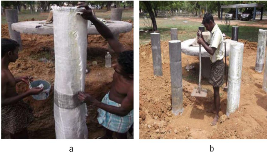
Figure 3.15. a. coting column GFRP wrapping b. Filling of excavated soil [34].
