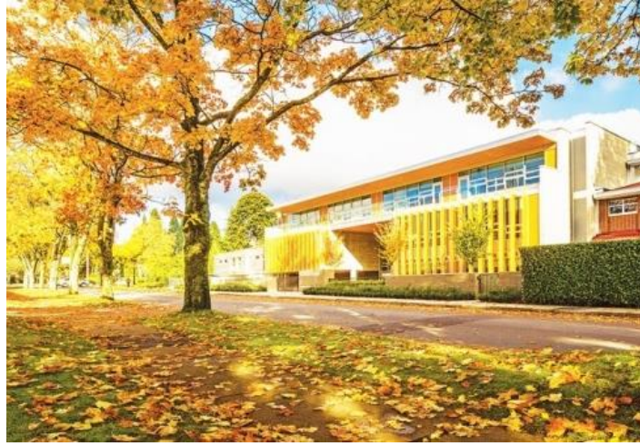
Şekil 2.4. York House Senior School, Vancouver, Kanada (İnternet, 5).
