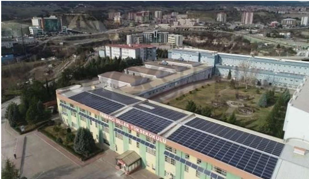
Figure 3.3. Installing PV system in Karabuk university.
