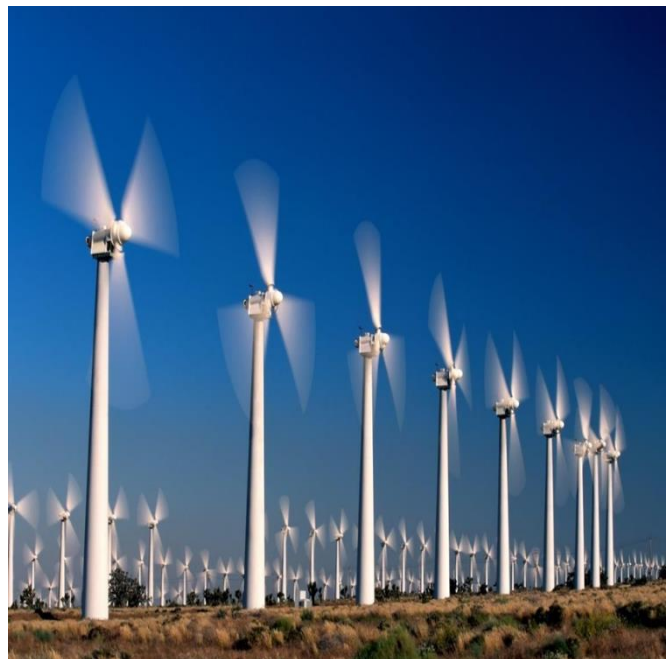
Figure 1.4. A modern wind farm [4].
