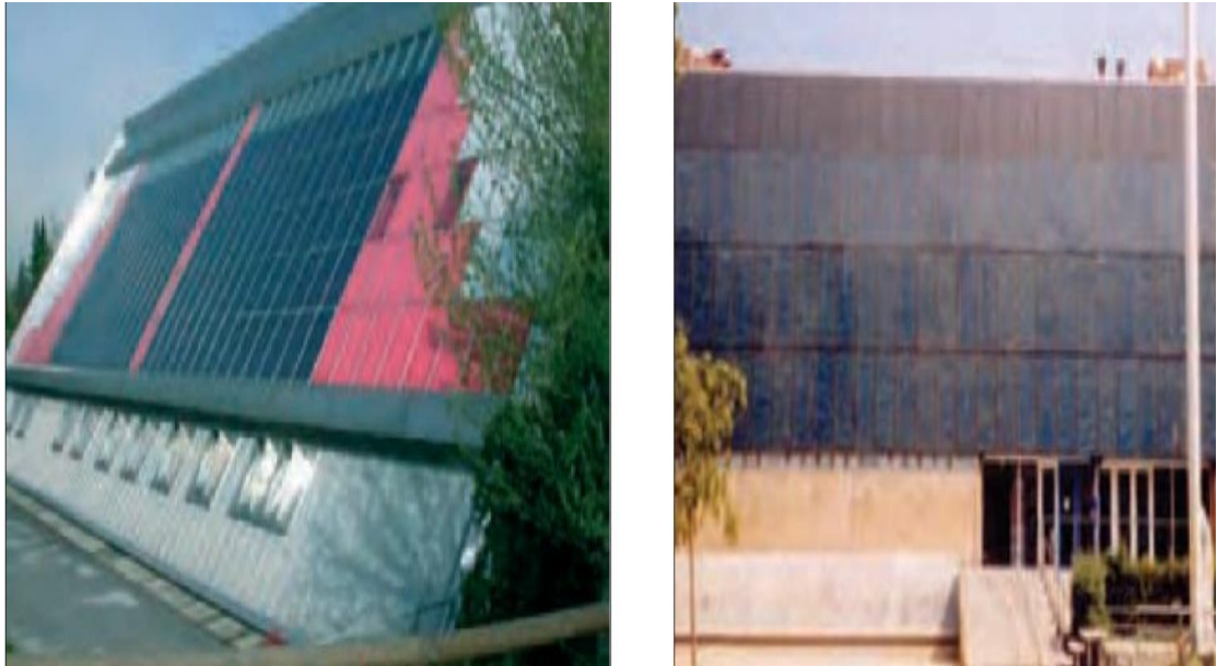
Figure 1.7. Solar cell ventilation collector with heat recovery on the facade of buildings [5].
