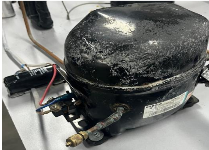
Figure 4.11. Low T (R404A) circuit Comp.
