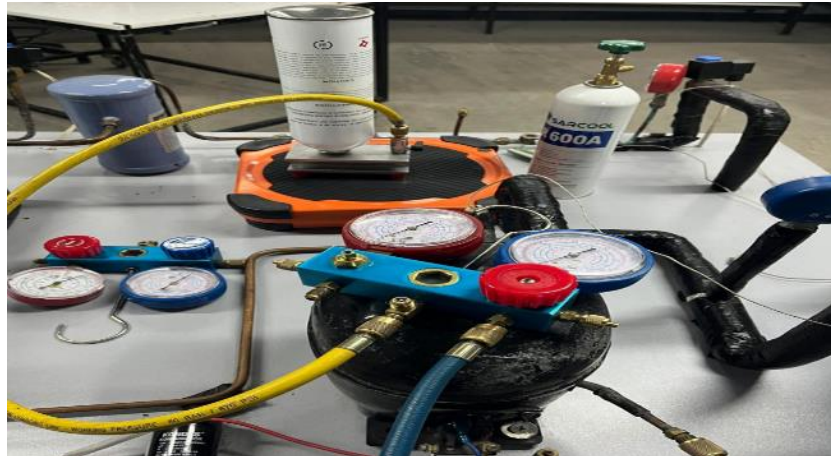
Figure 4.24. R600a refrigerant charging application.
