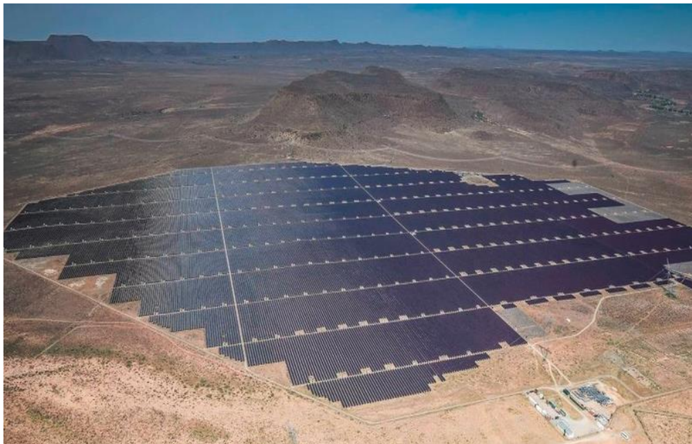
Figure 3.1. Photovoltaic (PV) solar power generation. Sudair /Saudi Arabia [81].
