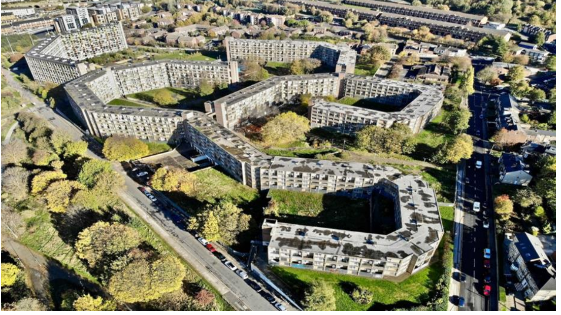
Şekil 2.4. 1961, Park Hill Development, Sheffield, ENGLAND, Sheffield City Architect [17]
