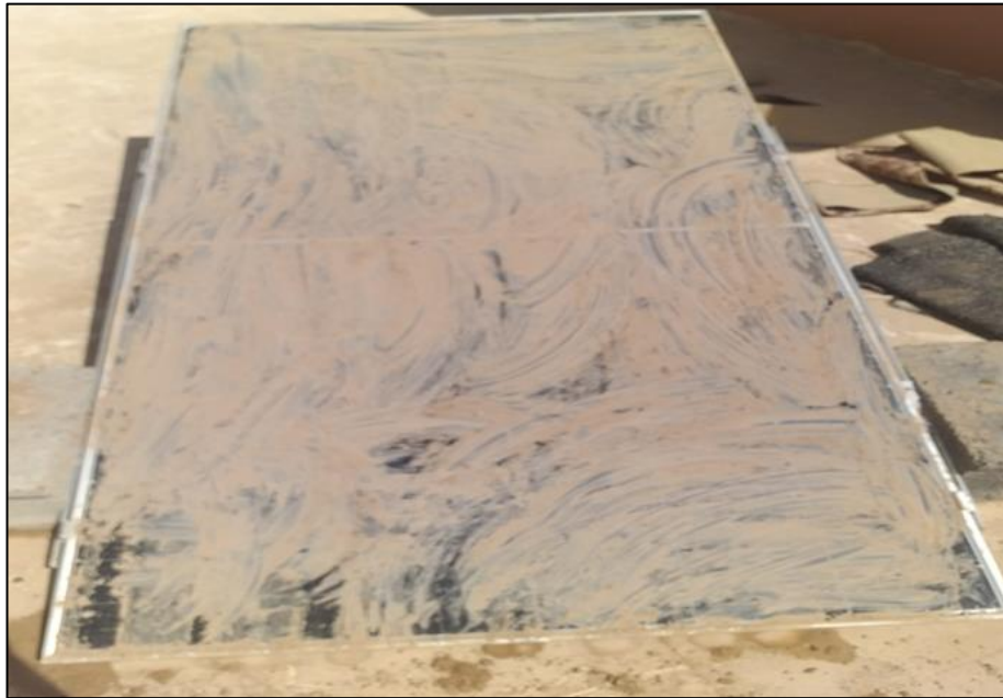
Figure 4.5. Large amount of dust deposits on the solar cell surface.
