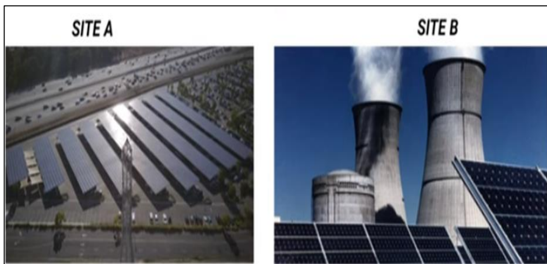
Figure 1.14. 1 MW same technology, same developer, same direction/azimuth [61]. Among both plants, which plant will give a higher output, higher efficiency, and a higher generation at the end of the month?
