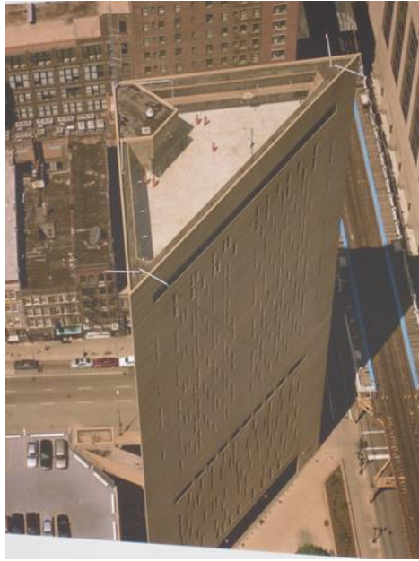
Şekil 3.35. 1975 Chicago, Metropolitan Correctional Center ( https://99percentinvisible.org/episode/episode-26-the-mcc-chicagos-jailhouse/ , 2023).
