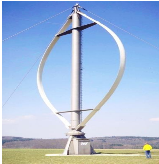
Figure 1.4. Darrieus Vertical Wind Turbine model [13].
