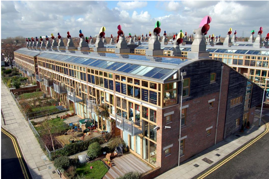
Figure 1.3. An example of zero heating building [91].
