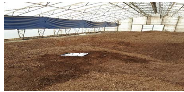
Figure 5. View of the greenhouse
