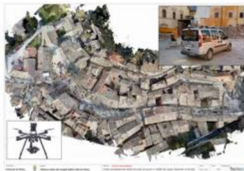
Figure 2. Damages in historical centre of Visso: Prospective views of point cloud in rgb by laser scanner and drone, 2017.
