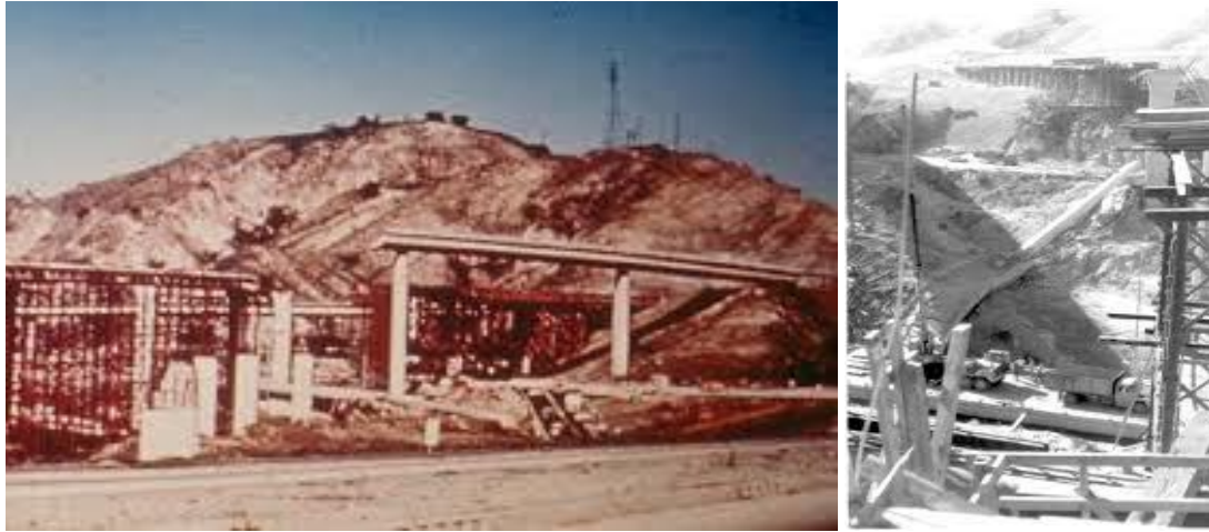
Figure 3. The collapsed sections of South Connector Overpassing after the San Fernando Earthquake [4]
