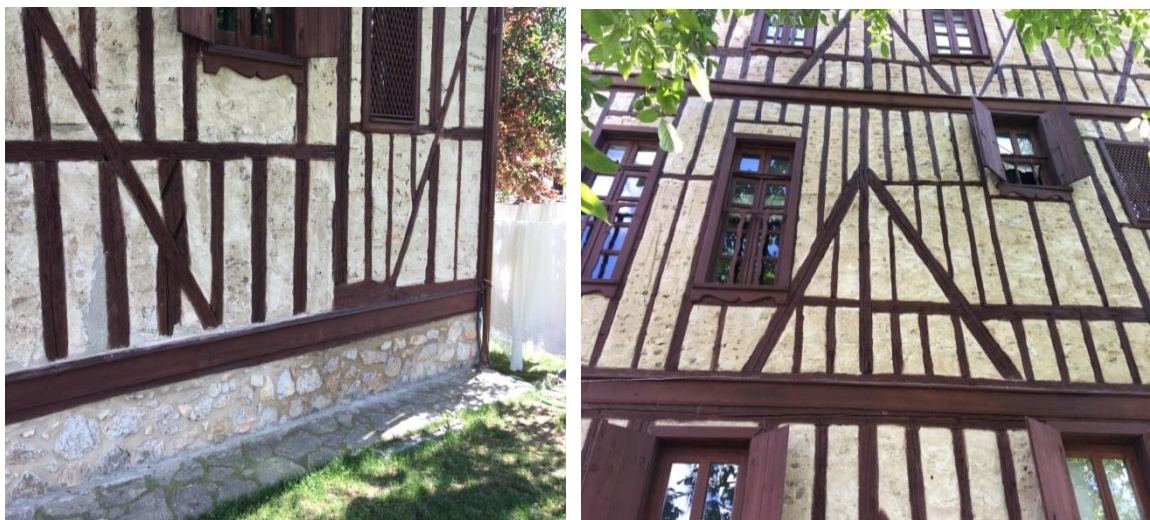
Figure 2. Brace types, 45 ° - 60 ° angle, support brace and V-cross.
