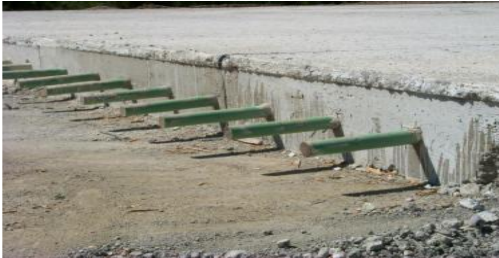
Figure 5.17. Construction joint [70].
