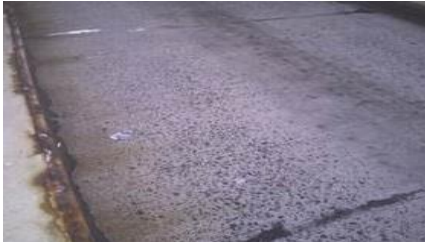
Figure 3.22. Polished aggregates [60].
