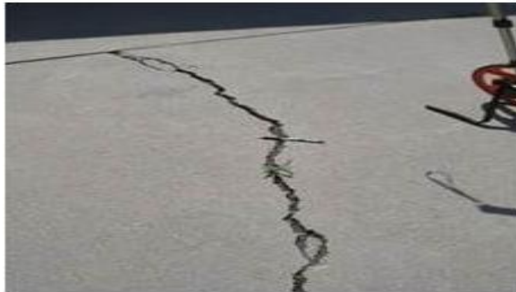
Figure 3.27. Linear cracking [60].
