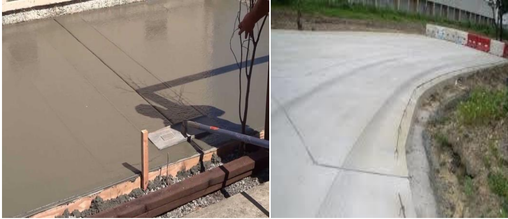
Figure 5.19. The joint between the concrete [63].
