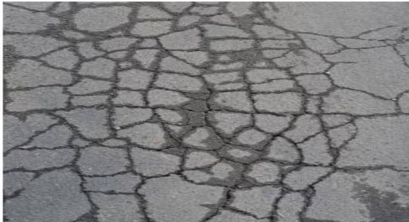
Figure 3.9. Alligator cracking [55].
