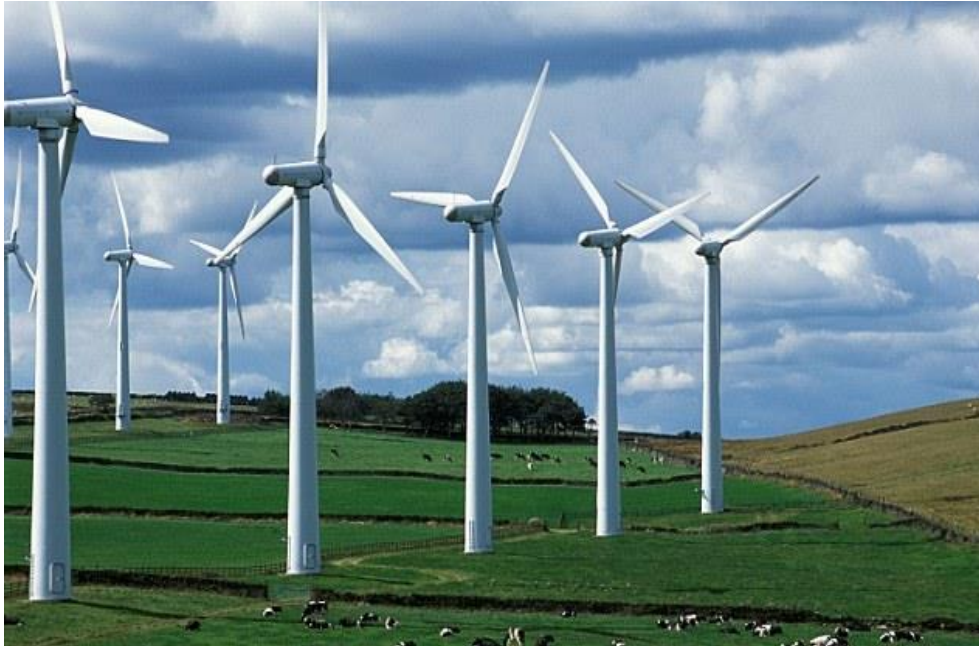
Fig. 1.1 Wind power plant station
