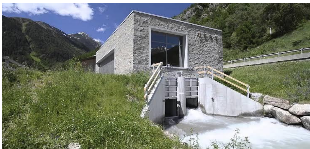
Fig. 1.2 Table Small Hydro generators – Susasca, Switzerland.
