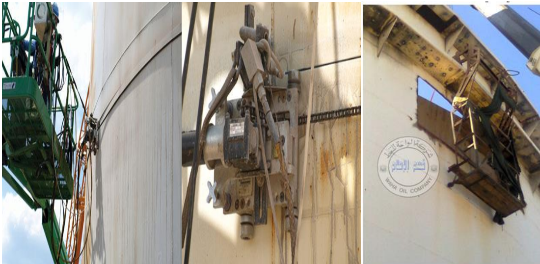
Figure 1.1. Cutting oil tank by AWJM [16].
